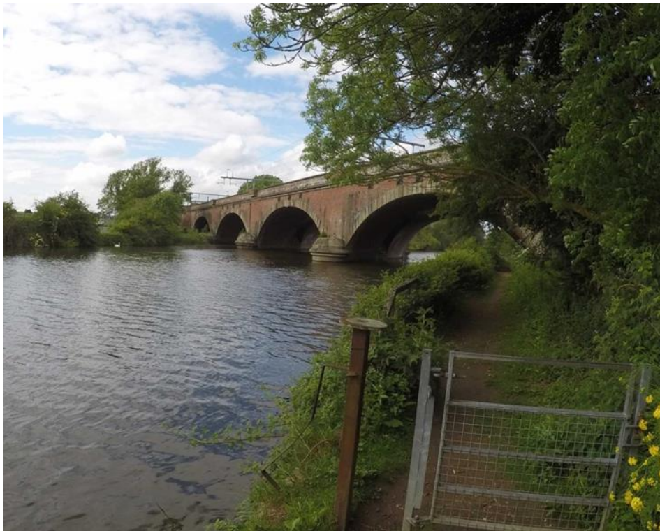
Photo 32: A four double-arched railway viaduct crossing the river Thames. Double = two four arched viaducts built next to each other with a small gap inbetween.
